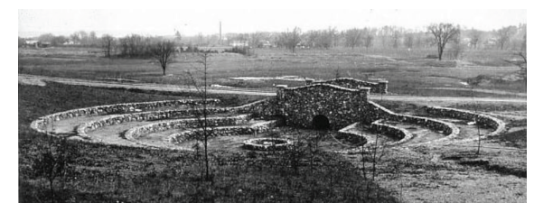
Originally built by the Works Progress Administration (WPA) in the 1930s as an erosion control pond.
