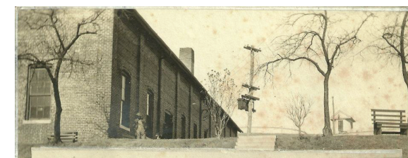
The waterworks include a 1899-1900 brick filter building with clerestories and 1915 addition, ca.1926-1936 brick chemical feed house.
